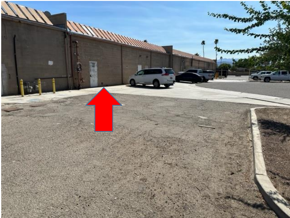
Rear View of Tenant Space
